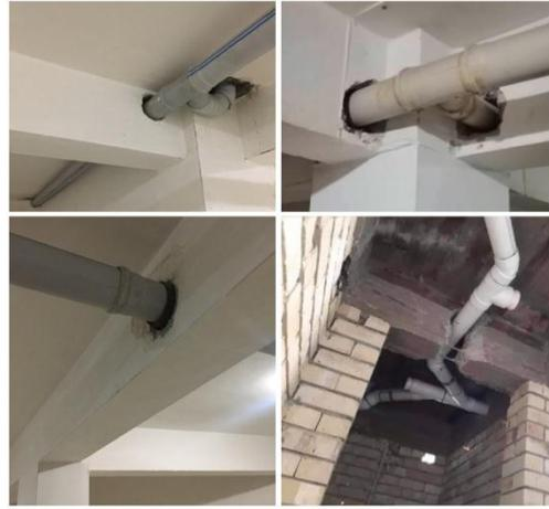
Fig. 1 Web openings in RC beams [11]
